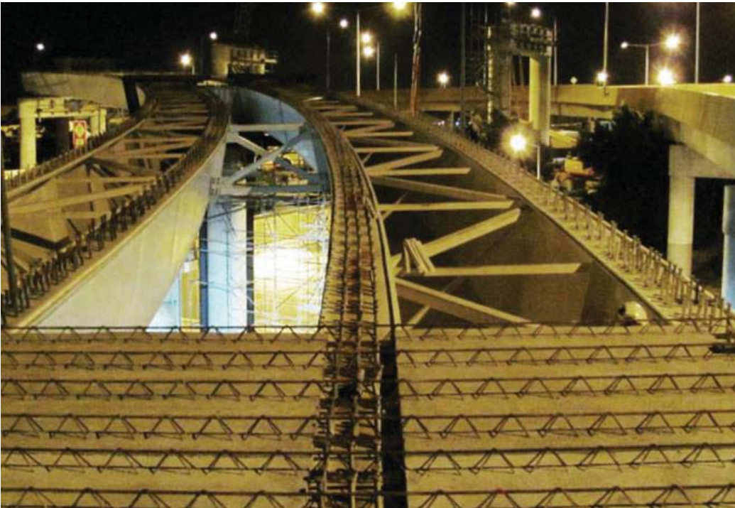
Figure 7.6 Humeslab being used on Airport Link in Brisbane
