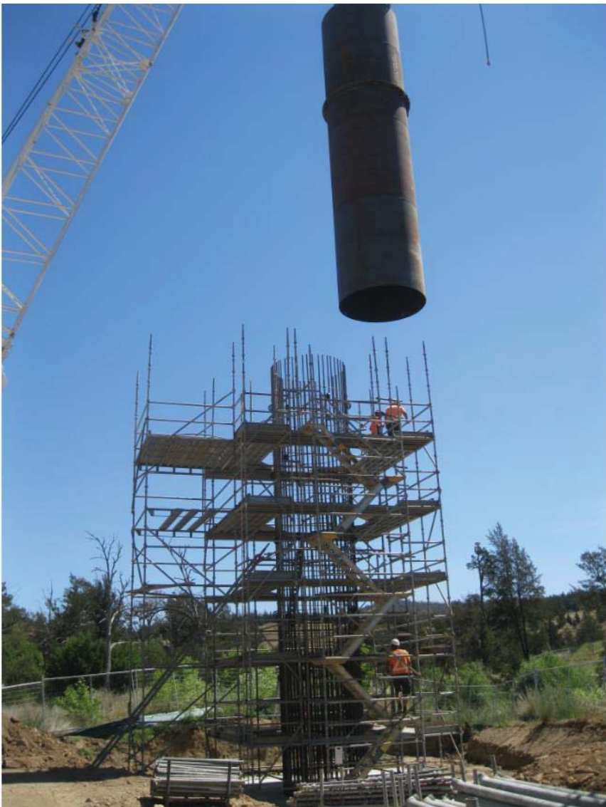
Figure 7.11 Butters Bridge Pier Construction
