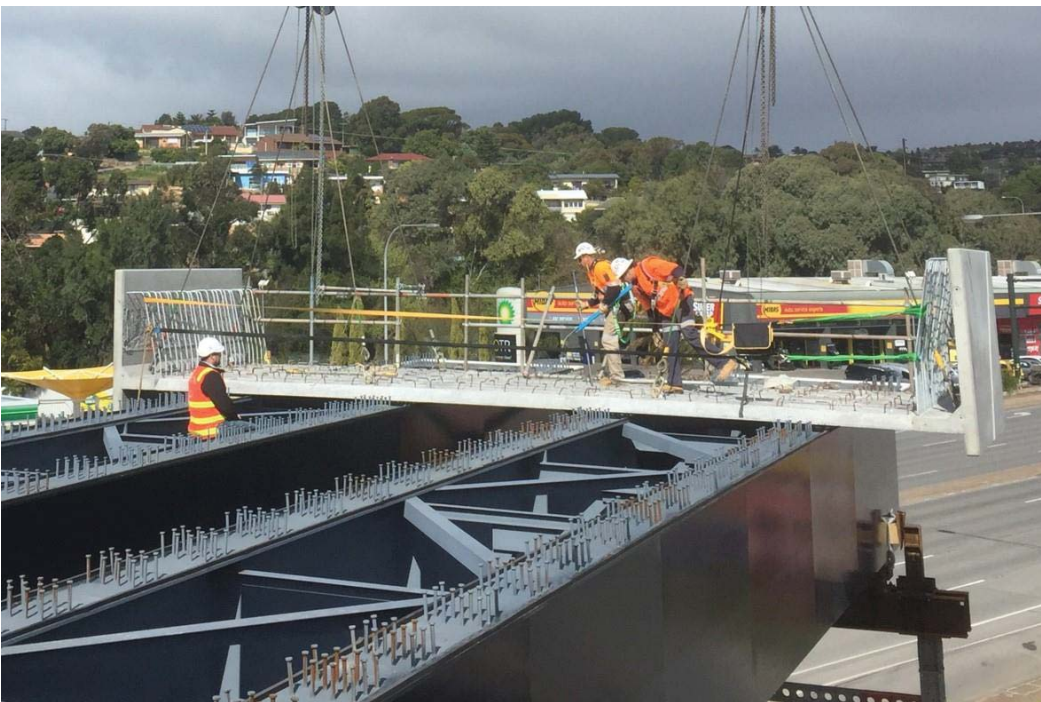
Figure 7.7 Bespoke decking system being used on the Darlington Upgrade in Adelaide.
