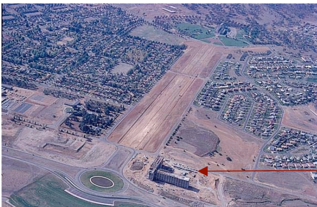
Figure 50. Aerial view of Anzac Parade looking North, under construction, c1965
