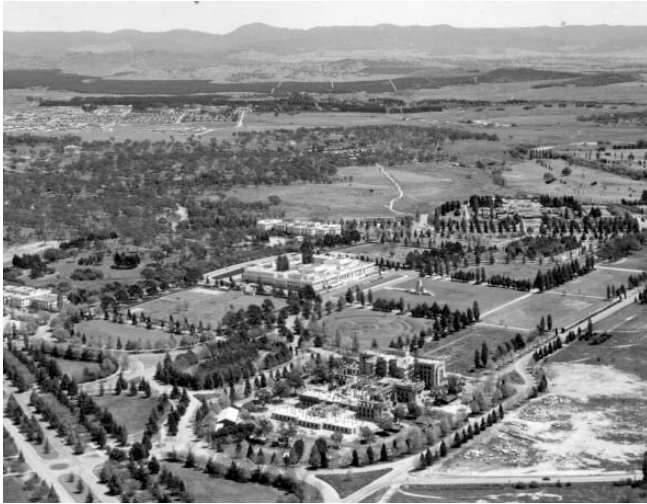
Figure 41. Parliamentary Zone South of the lake (not yet constructed) in 1953
