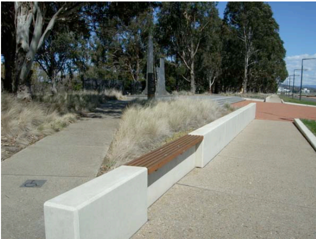
Figure 27. Typical concrete and timber seat on Anzac Parade with the RAAF Memorial in the background Source: Duncan Marshall
