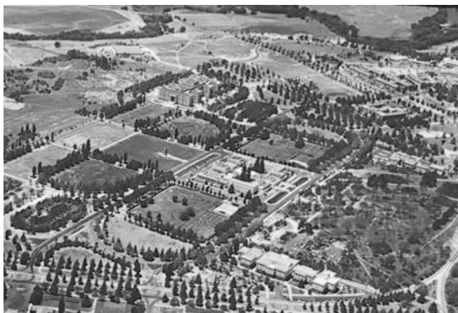
Figure 44. Parliamentary Zone South of the lake (not yet constructed) in 1958
