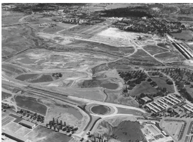
Figure 48. View South over Molonglo floodplain during construction works for lake, 1963
