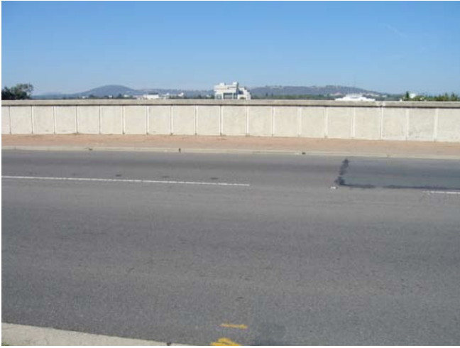
Figure 81. View south along Land Axis from Parkes Way Source: Craig Burton 2006
